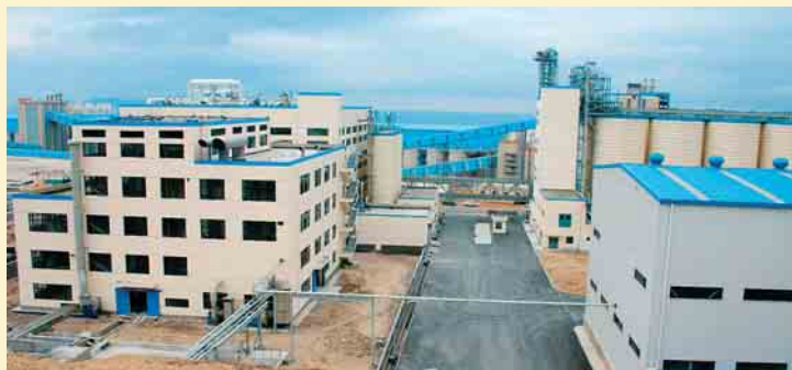
Dalian Nisshin Oil Mills, No. 2 Plant The No. 2 plant operated by Dalian Nisshin Oil Mills, Ltd. came on stream in March 2005
