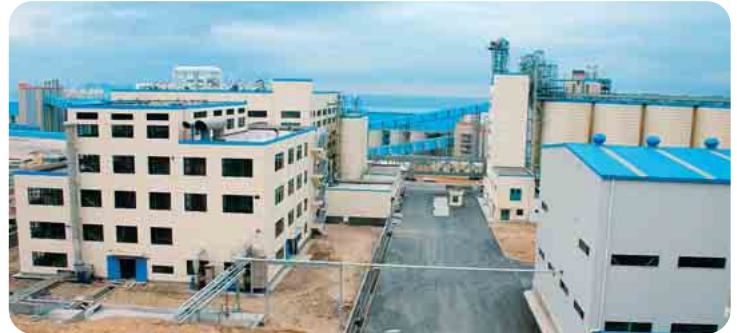
Dalian Nisshin Oil Mills, New Plant The new plant operated by Dalian Nisshin Oil Mills, Ltd. came onstream in March 2005
